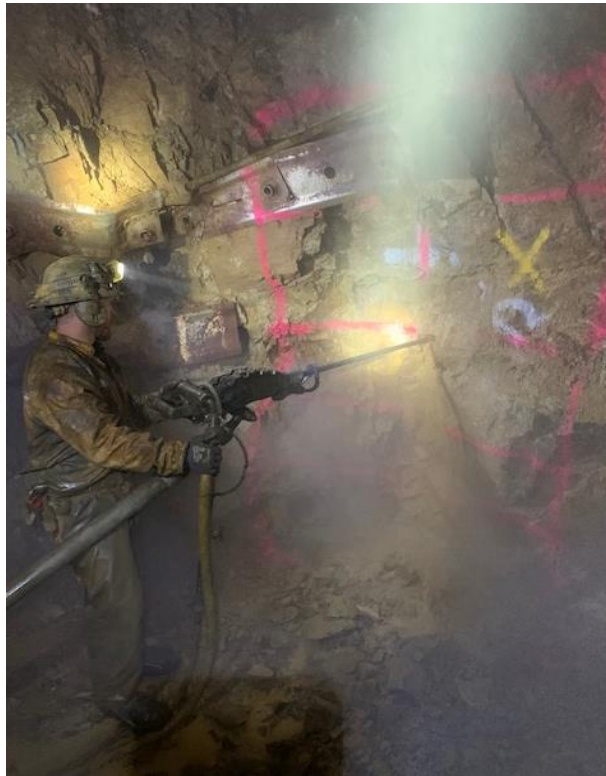
Figure 2: Underground drilling underway to establish new drill bay at Silver Strand
